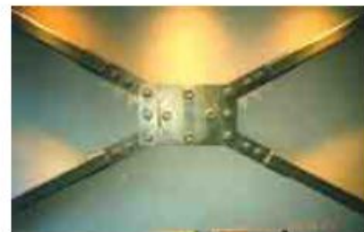
Friction Damper in Tension-only Cross Brace
