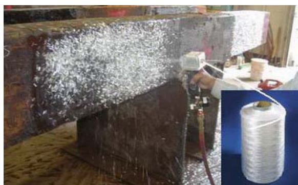
Spraying Fiber on the Wet Surface
