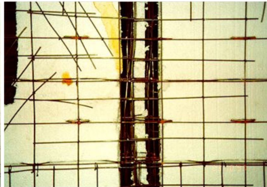
Connection of Three Walls
