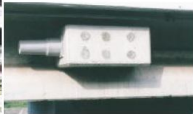
View of anchorage block showing position of 6 AFRP tendons.
