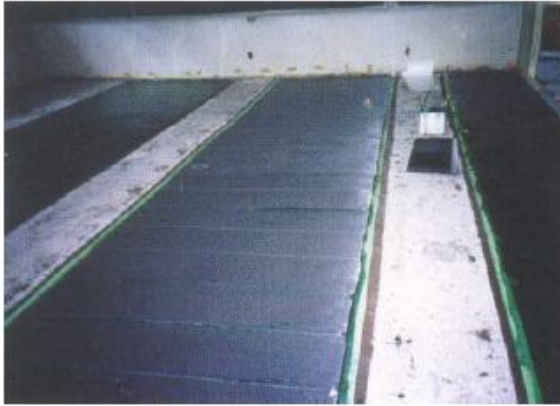
(a) repair of cracked floor
