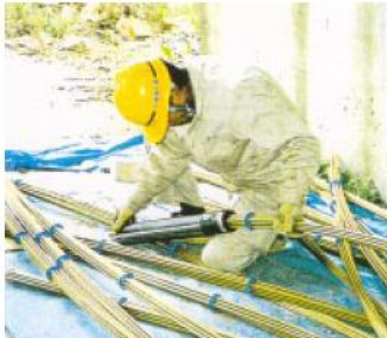
Preparing the anchorage (bond-type)
