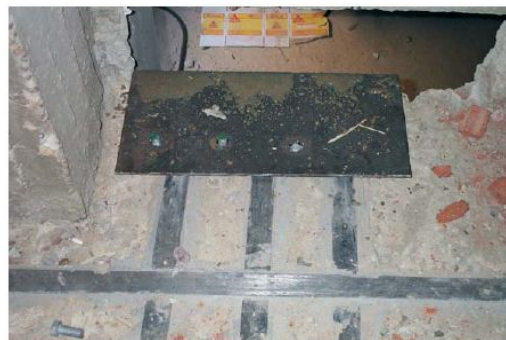
Mechanical Anchorage of CFRP plates
