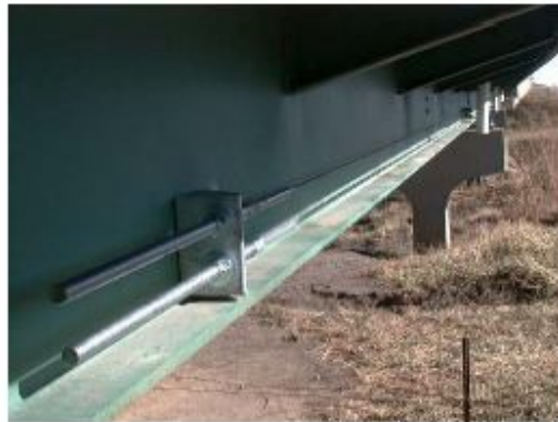
CFRP Rods on span
