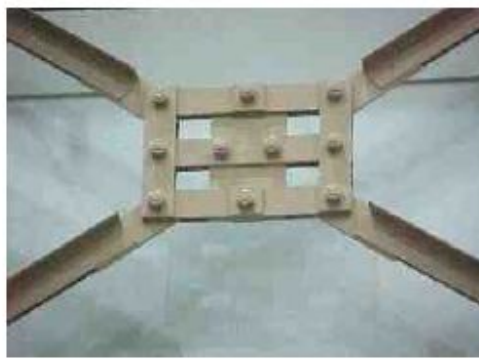
Cross Brace Pall Friction Damper
