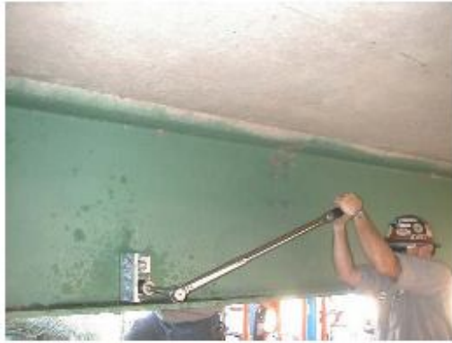
(a) Installation of anchorage assembly
