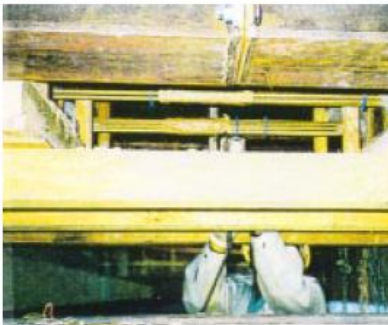
Cutting of tendons between girders after cure of concrete in anchor blocks.
