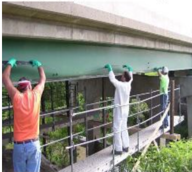
(e) Placement of CFRP plate
