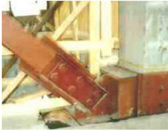
Pall Friction Damper
