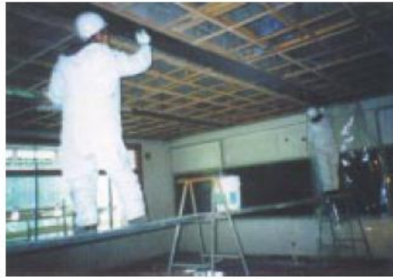
(b) repair of slabs
