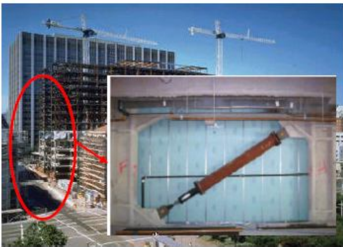
Viscous dampers in steel framed building.
