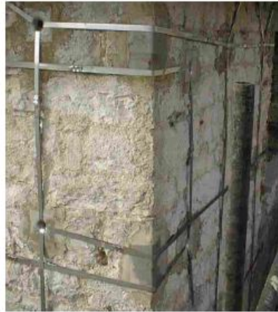
Detail of the connection between orthogonal walls.
