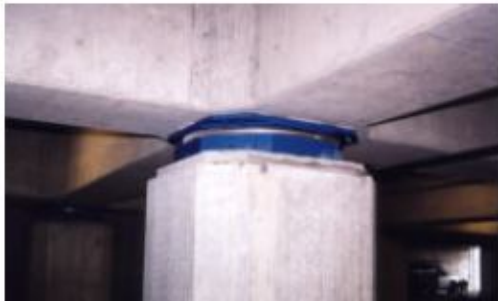
Installed Bearing, Hayward City Hall
