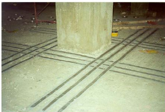
CFRP strips attached to the top surface of concrete
