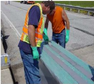
(c) Epoxy application on CFRP plates
