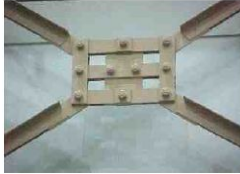
Cross Brace Pall Friction Damper
