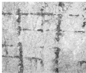
Corrosion of the net
