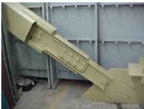
In-line Pall Friction Damper
