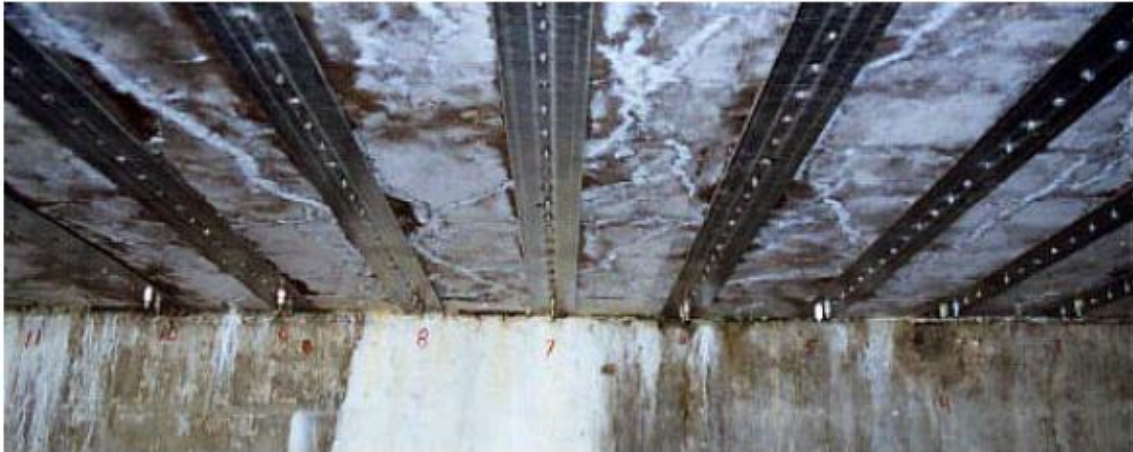
12 in. Strip spacing between FRP strips
