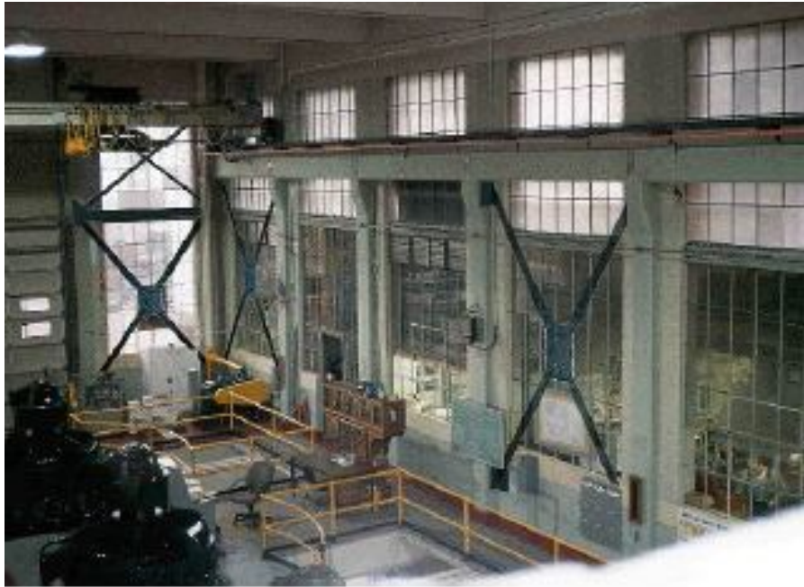
Pump House building: rendering of installation of friction dampers
