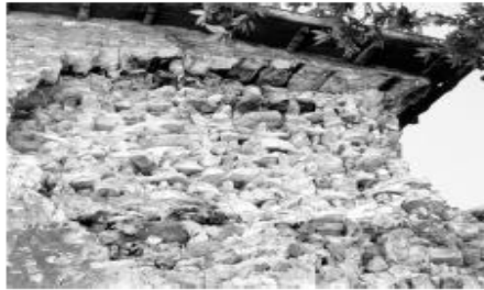
Separation of the two leaves of a wall
