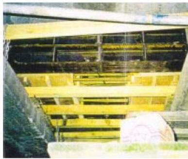
Placement of temporary reaction devices between girders.
