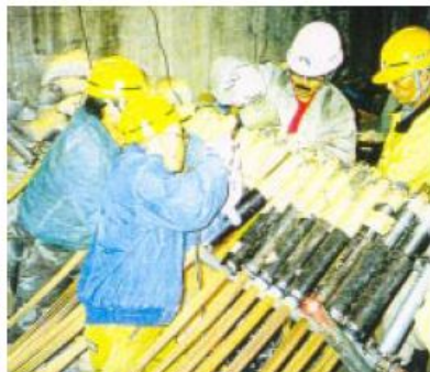
Injection of mortar into the tendon mounted anchorages.
