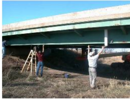
(b) Placement of CFRP rod
