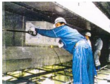
Installation and jacking of external steel cables.
