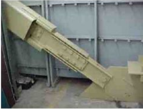
In-line Pall Friction Damper
