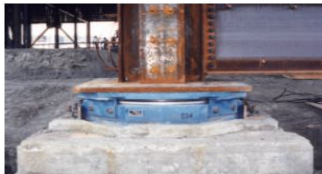
San Francisco Airport Bearing Installation
