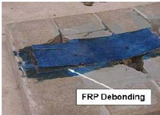
(a) FRP Debonding
