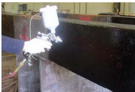
Spraying Resin to Wet out the Surface
