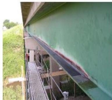
(f) CFRP plate installed.
