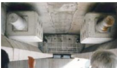
End view of anchor blocks with external cables and anchorages.
