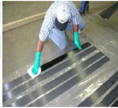
(b) Cleaning CFRP plates
