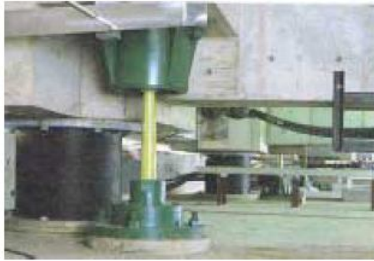
Steel rod damper combined with a NRB
