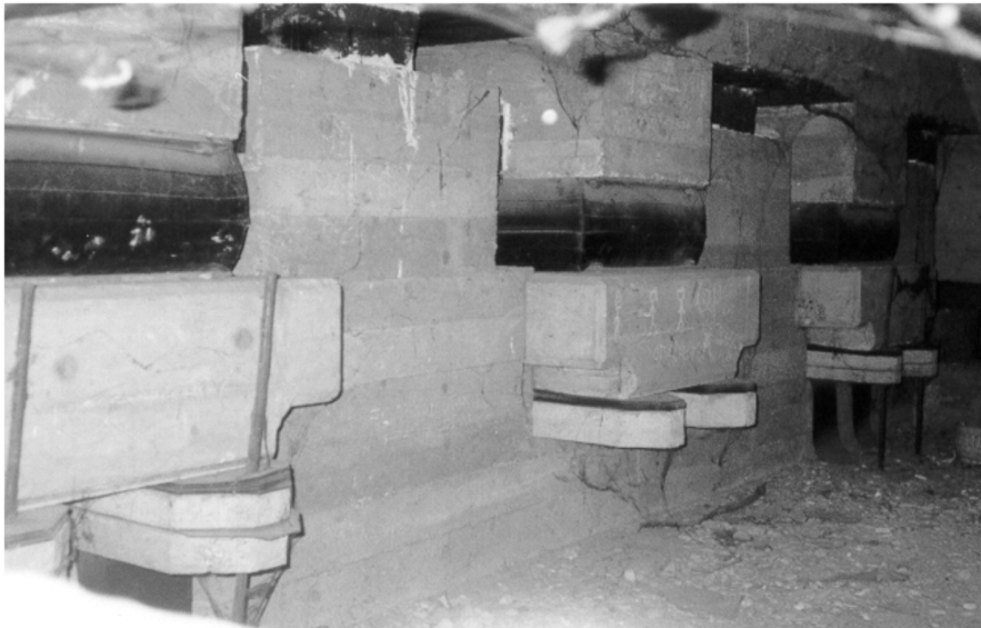
Rubber bearings placed between the strip foundation and the building
