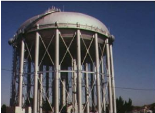
Elevation of retrofitted tank
