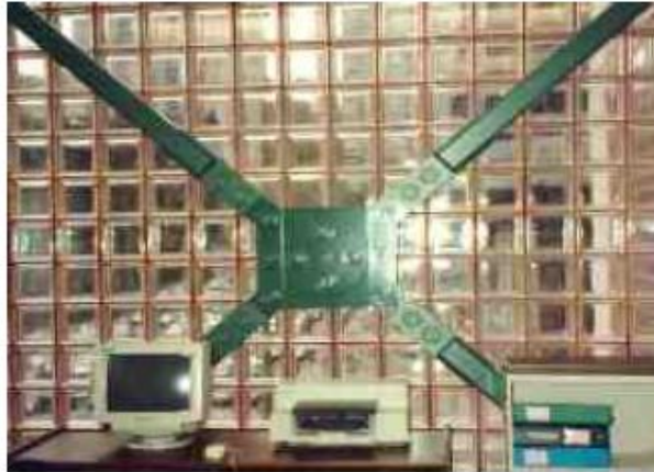
Pall Friction Damper in Cross Bracing
