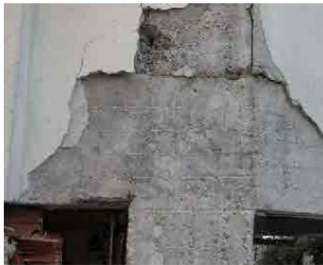
Visibly narrow shear crack and flexural crack occur in beam. No shear cracks are observed in the beam-column joint.
